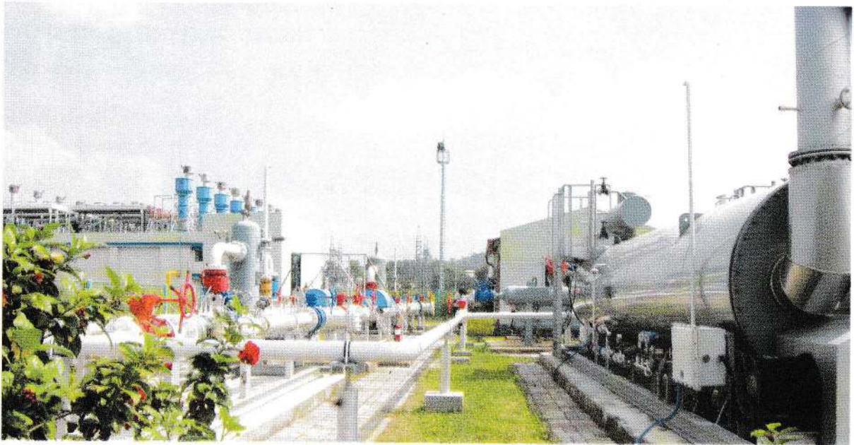
Partial view of RMS of 86MW Shahjibazar Power Company Ltd. Habiganj
